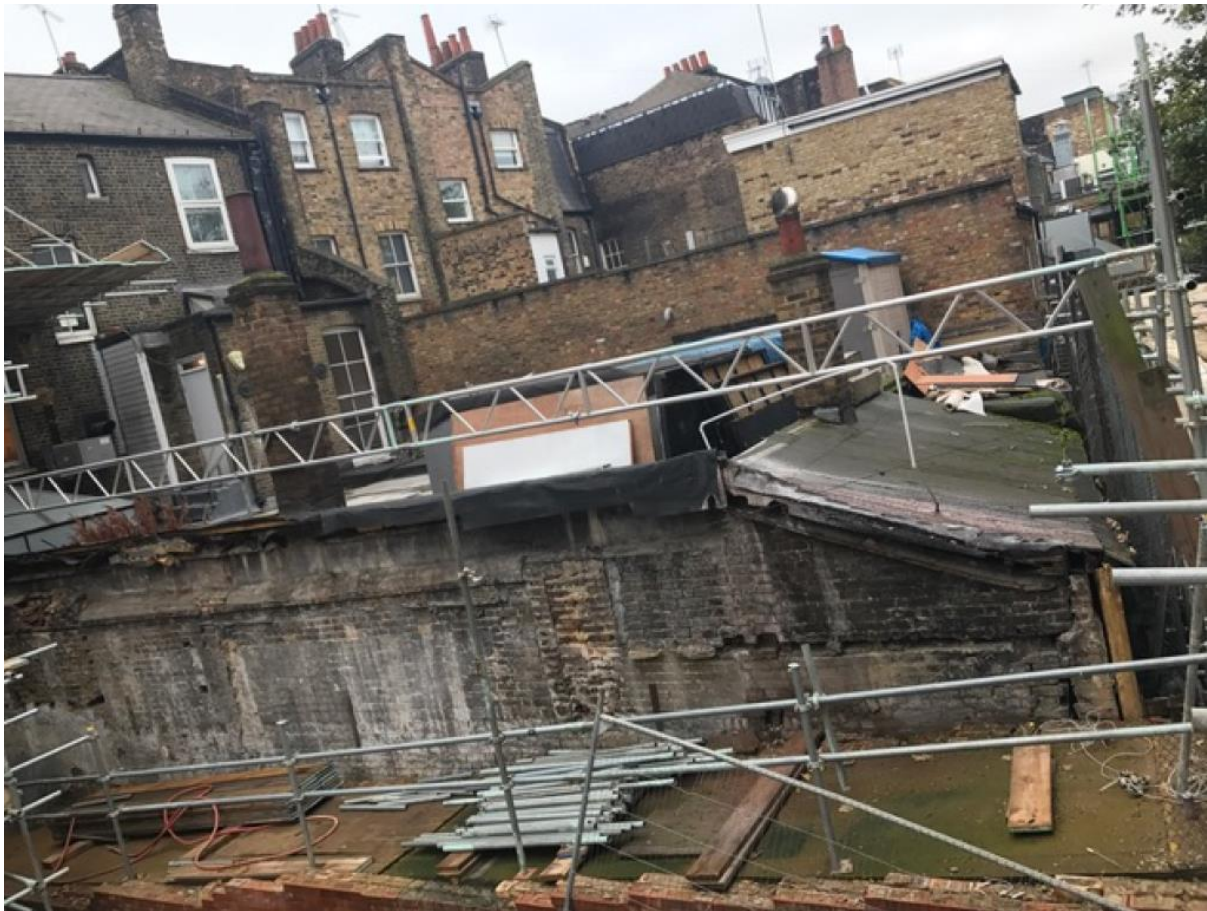
Figure 6: Kings Head lean-to extension to be demolished.
