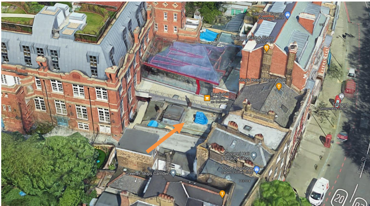
Figure 5: View looking onto rear roof of Kings Head public house
